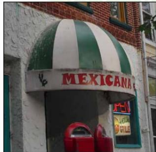
Inappropriate Awning Scale
